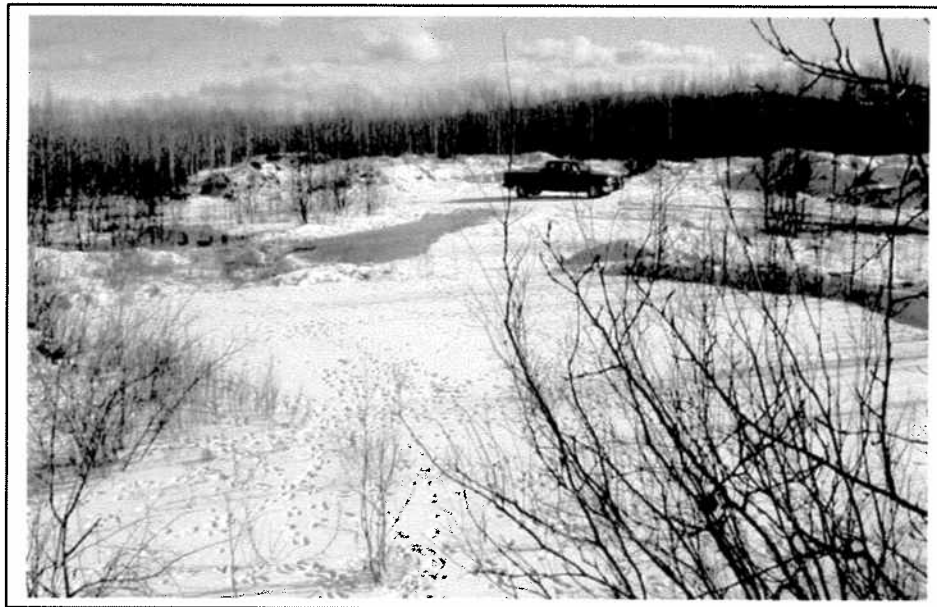
Fig 1: Septage Disposal Pit with Overflow
