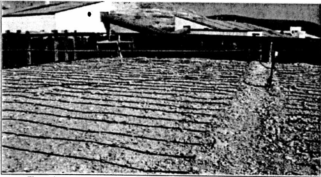
Figure 2: Rows of flexible plastic tubes with drip emitters used to apply the leaching/rinsing/neutralizing solutions on top of the ore.
